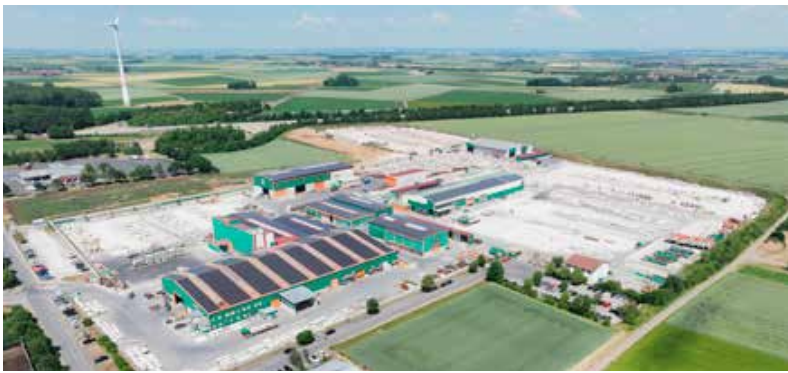
Bird's eye view of the Weber concrete plant in Ippenheim
